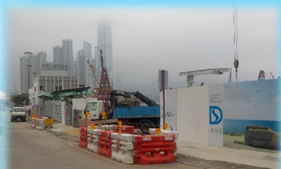
海輝道工地入口 Site Entrance at Hoi Fai Road
