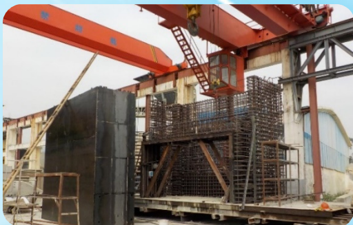
在工場製預製組件 Constructing pre-fabricated concrete modules at precast yard
