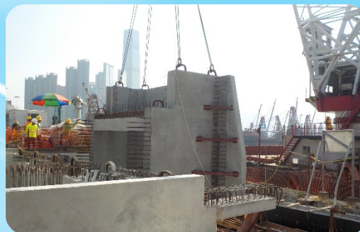
正在工地進行安裝 Installing prefabricated concrete modules on site
